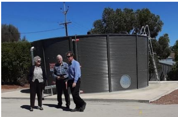
Photo of Laurel Jared, Geoff Beaty & Works Supervisor inspecting the new tank
